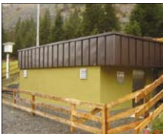
Pumpstation Neurur (Foto: Venier)
